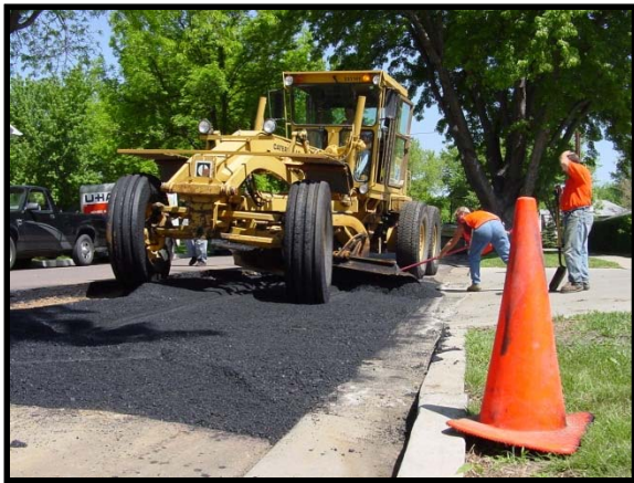
Overlay & Concrete Pavement Restoration $44.5M
